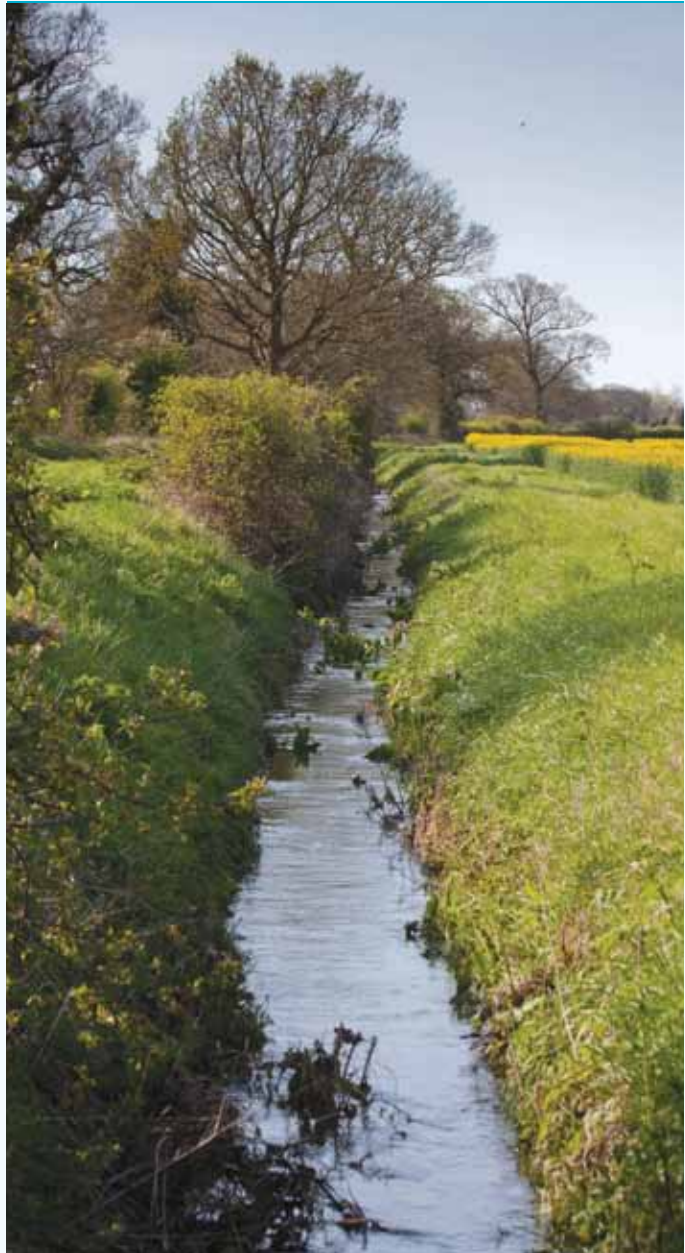
In its upper reaches the river channel has been modified into a network of deeply-incised ditches. This has not only reduced the ability of that land to retain and slowly release water, but has created a considerable problem of soil erosion and sediment loading.
