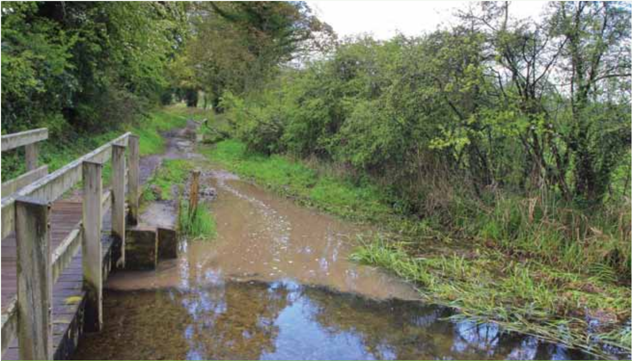
West Acre ford after a heavy downpour May 2012: a clear illustration of the impact of point-source sediment pollution. Diverting this flow into a wetland settlement pond in the meadow beside the river would make a big difference with the add-on ecological benefit of creating more wetland habitat.
